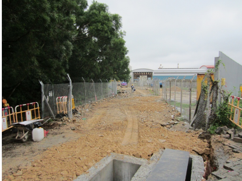
Photo 1 – For the completed section of land duct, excavated materials have been backfilled and the site has been reinstated to its original status.
