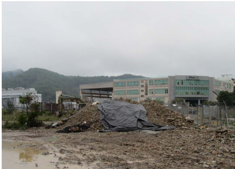
Photo 2 – Some stockpiles of the excavated soils from the new beach manhole and land duct were partly exposed in the rain.
